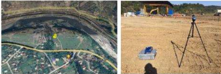
Figure 5-9 Point N3 KM 5.8
