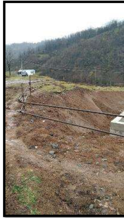
Photo 3. Concrete Plant №1 and Camp №3: Good Observation: Excavation area has been enclosed with protective guardrails;
