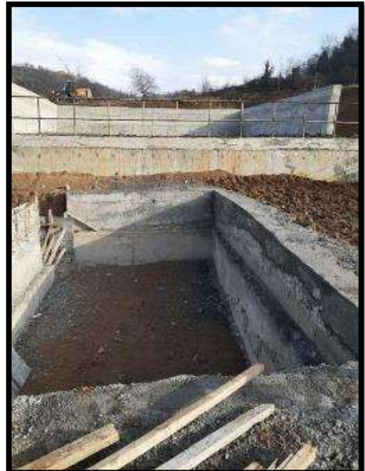
Photo 1. Concrete Plant №1: Non-Conformance: Excavated area/opening must be enclosed with protective guardrails;
