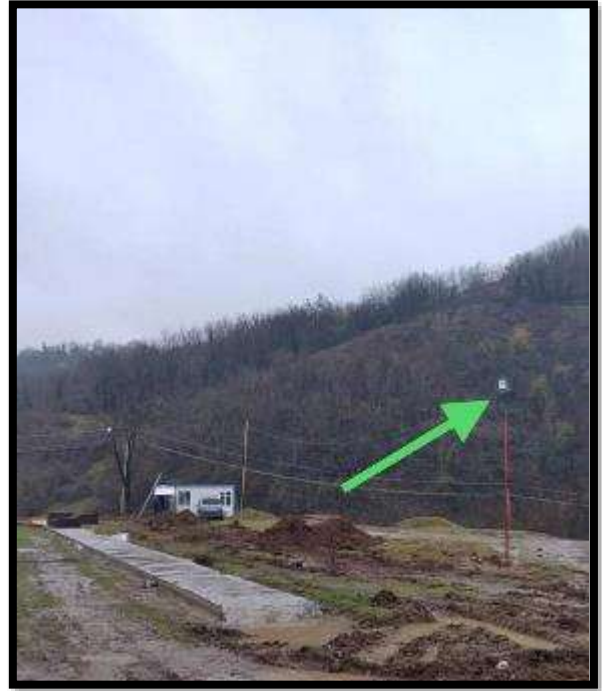
Photo 2. Concrete Plant №1 and Camp №3: Good Observation: Camp territory is appropriately illuminated;
