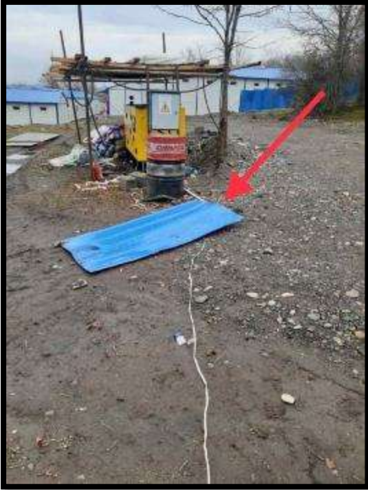
Photo 1. Camp №6: Non-Conformance: Electrical cable is placed on the wet ground and also sharp piece of metal plate is placed on top;
