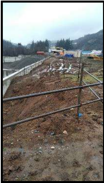
Photo 3. Concrete Plant №1 and Camp №3: Good Observation: Excavation area has been enclosed with protective guardrails;
