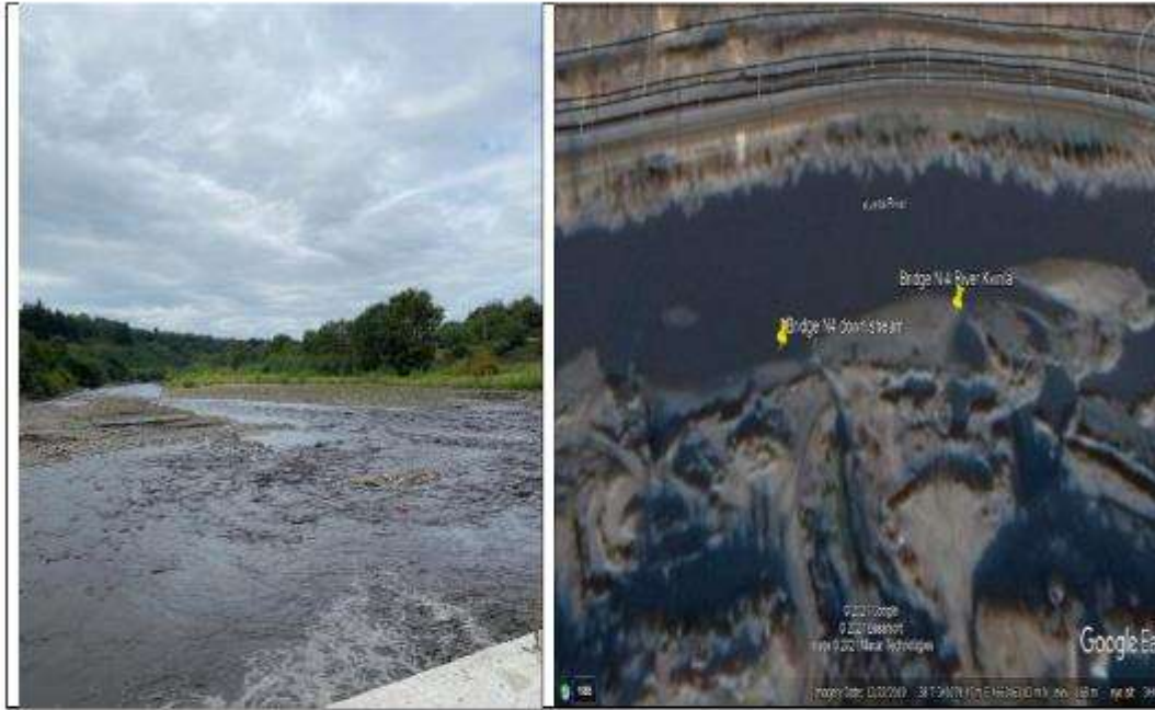
Figure 5-2 Bridge N4 downstream (Kvirilla river)
