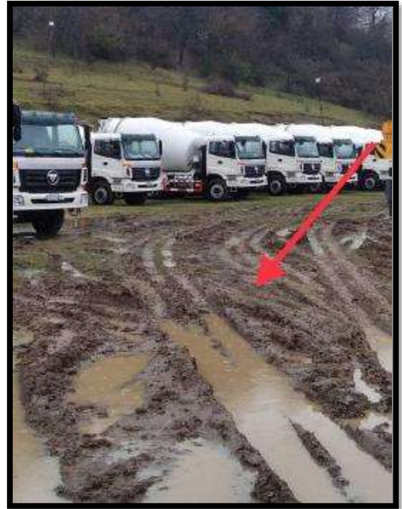
Photo 5. Concrete Plant №1 and Camp №3: Non-Conformance: Territory used for heavy machinery parking must be graveled;
