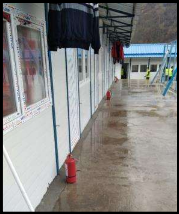
Photo 4. Concrete Plant №1 and Camp №3: Non-Conformance: Fire extinguishers must be placed in special, protective boxes;
