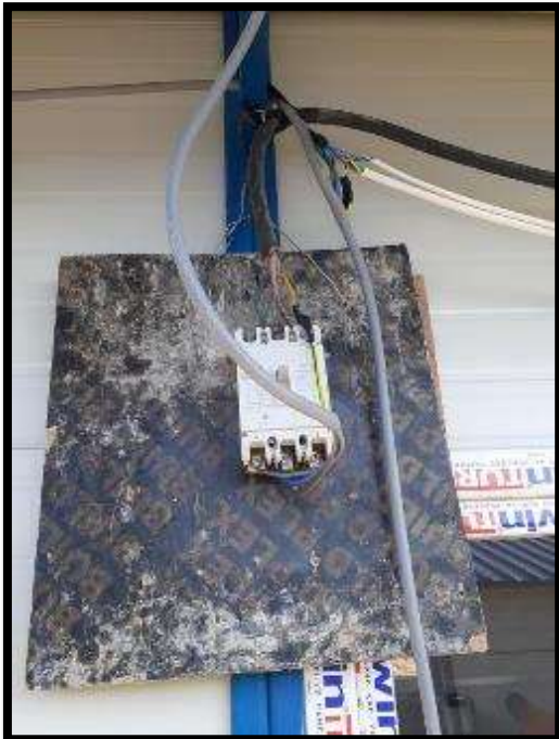
Photo 2. Camp №6: Non-Conformance: Electrical switches and relays must be put in a special box. Box must have lock and safety sign;
