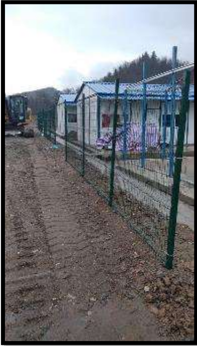
Photo 1. Concrete Plant №1 and Camp №3: Good Observation: Accommodation camp fencing procedure is in the progress;
