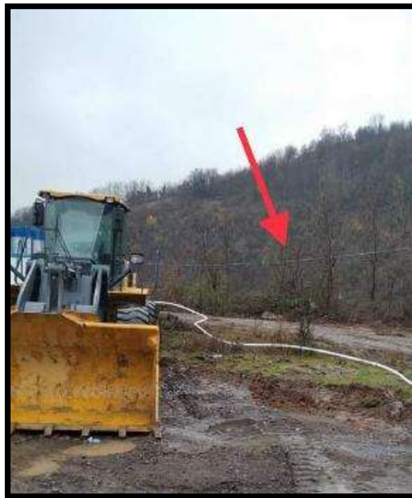
Photo 6. Concrete Plant №1 and Camp №3: Non-Conformance: Electrical cable must be raised at appropriate, safe height;
