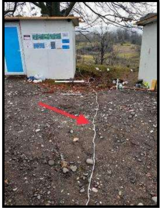
Photo 1. Camp №6: Non-Conformance: Electrical cable is placed on the wet ground and also sharp piece of metal plate is placed on top;
